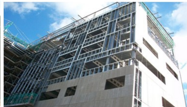
4. shear walls with gypsum sheathing
