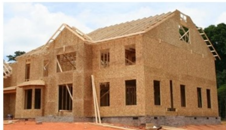
3. shear walls with wood sheathing
