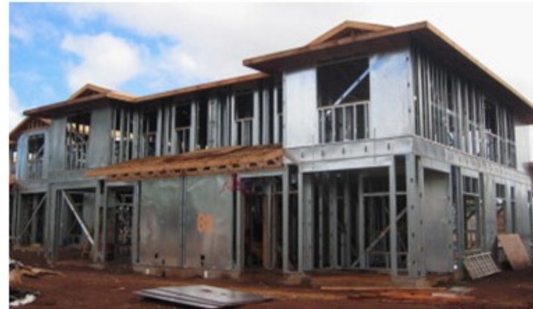
2. shear walls with steel sheet sheathing
