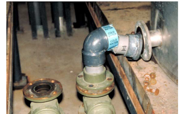
NISEE, University of California, Berkeley PEER Center, Edgumbe Collection No. ED34
