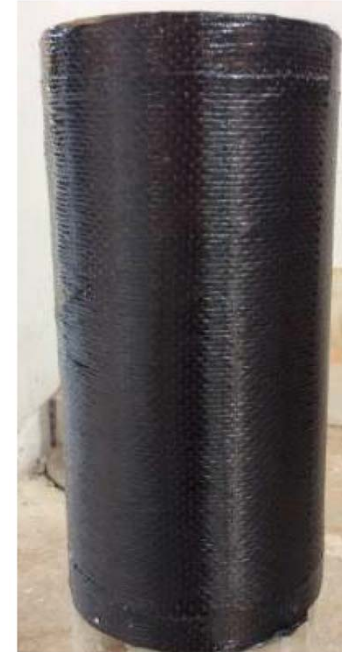
confinement through FRP jacket or strips
