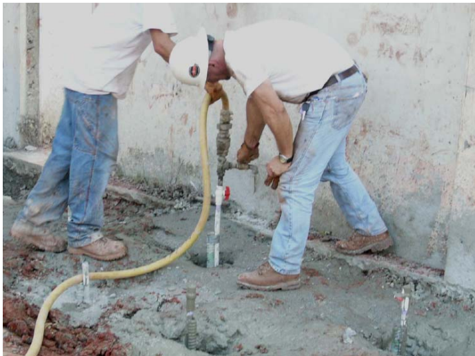
addition of micropiles to footing foundation
