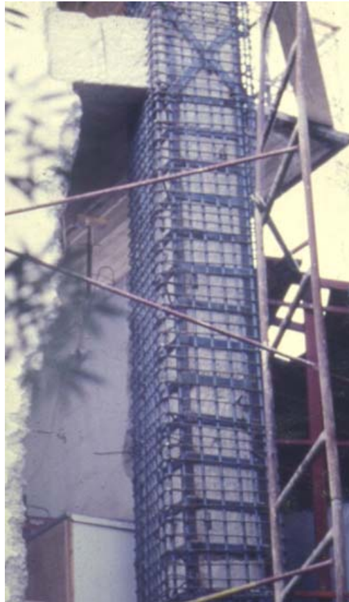
confinement through steel cage
