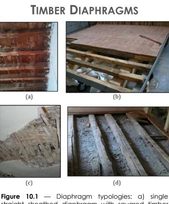
**Figure 10.1** — Diaphragm typologies: a) single straight sheathed diaphragm with squared timber joists; b) floor with clay tiles over joists; c)/d) floor built with the so-called "malta-paglia" (mortar-straw) technique, beneath and above views
