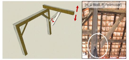
Loss of contact surface in a single-step joint (2006 Yogyakarta earthquake)
